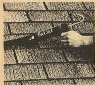
ASPHALT ROOF CEMENT
